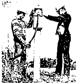
▲ PD-135 with special chuck drives 4" x 6" guard rail post
