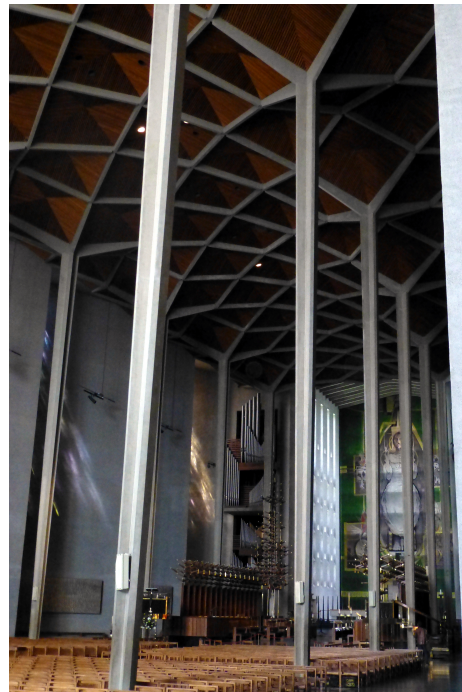
(b) Nave interior with pretensioned columns
