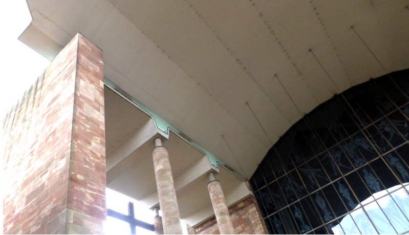
Figure 6: Underside of porch vault, showing the wires attached to West Screen
