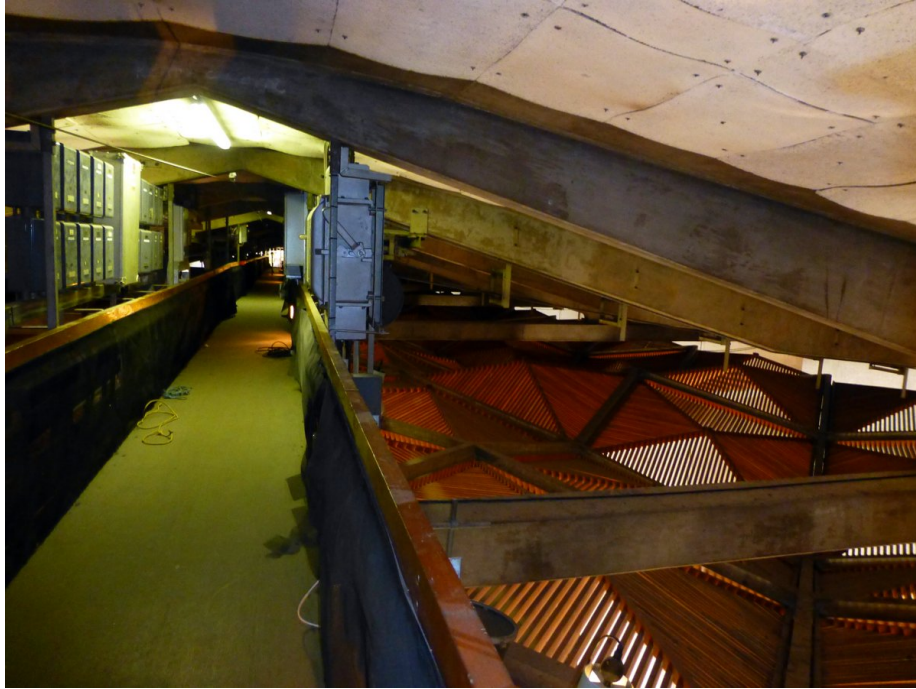
Figure 8: Nave roof seen from catwalk above tie beams
