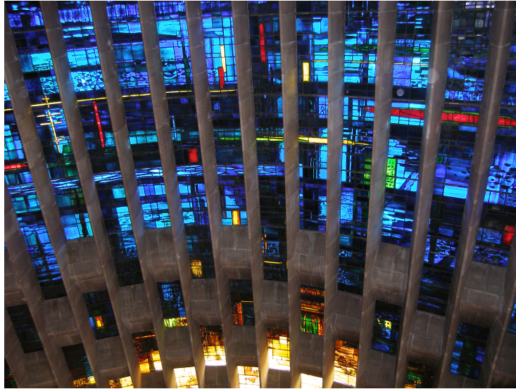
(a) Concrete mullions in Baptistry window
