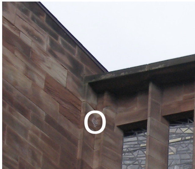
(b) Approximate location of tie beam anchor as viewed from outside
