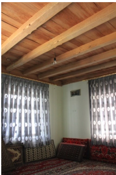
Figure 8.75: Internal wooden ceiling
