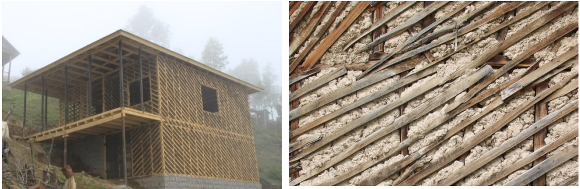
Figure 8.74: Two pictures of a house constructed with timber frame (wattle and daub or larde ) technology.
