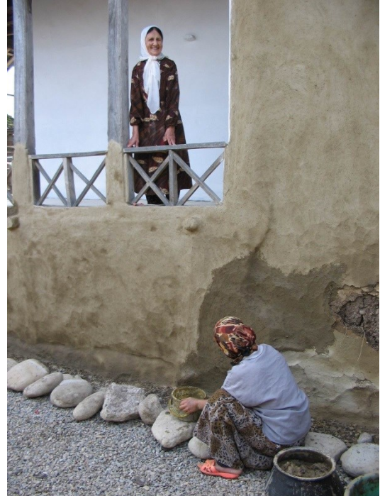
Figure 8.77: The woman repairing the external coat of a timber frame wall with mud mortar. Maintenance and reparation of vernacular house is of female responsibility.
