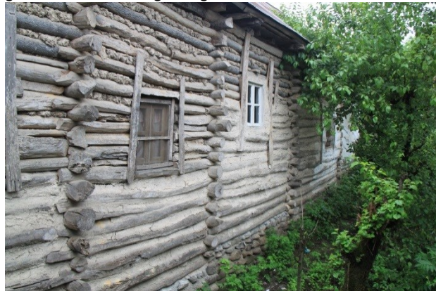
Figure 8.71: Detail of log on log wall of the vernacular house
