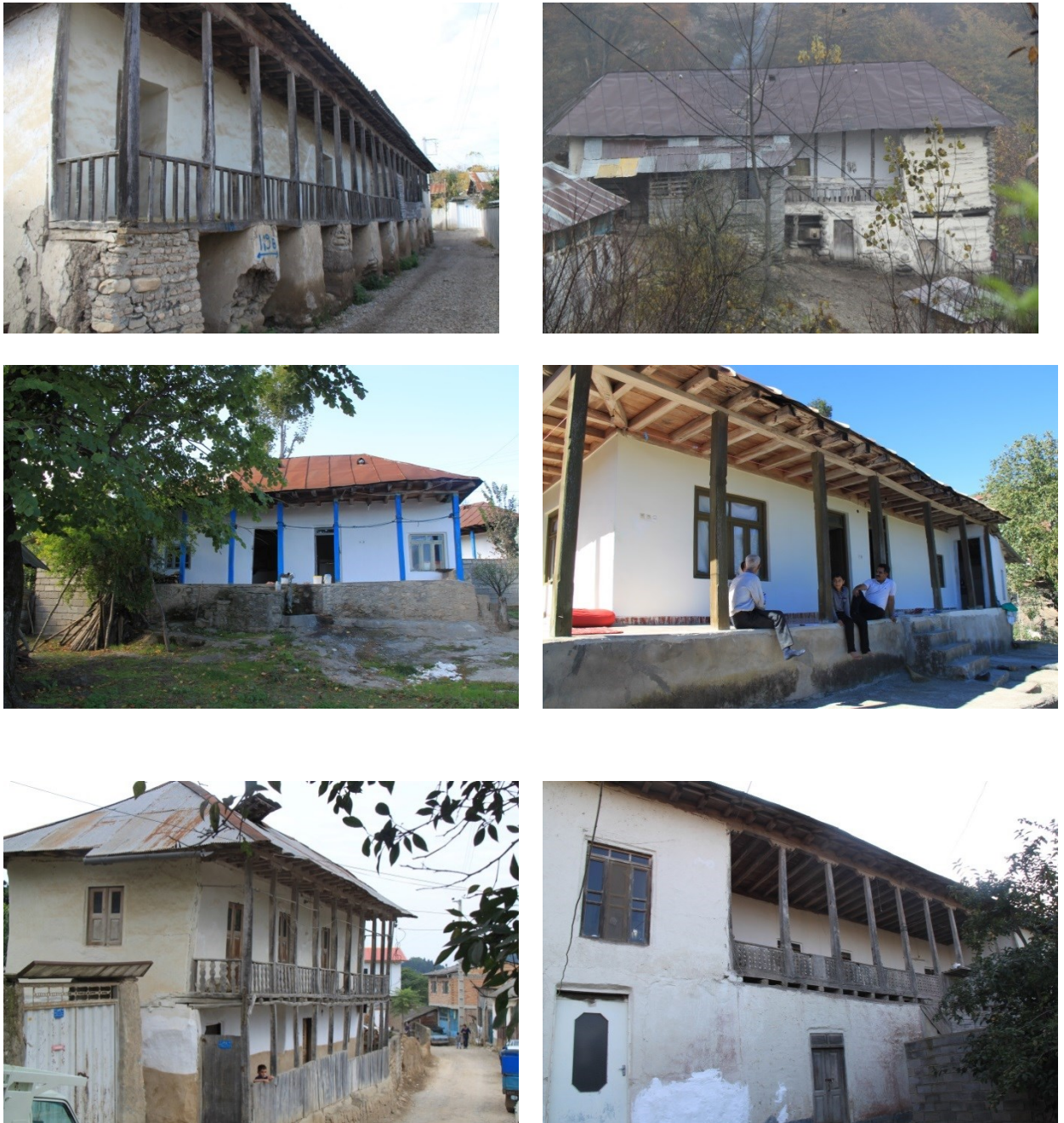
Figure 8.36: Pictures of some different types of vernacular houses within four villages of the region of this study
