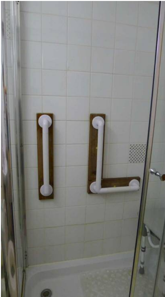
Figure 3: Grab rails installed in shower Photograph 4. Shower seat
