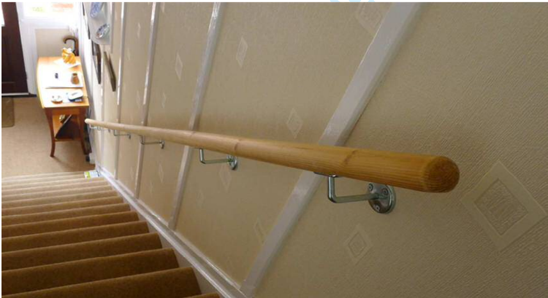
Figure 6. Banister installed along the stairs
