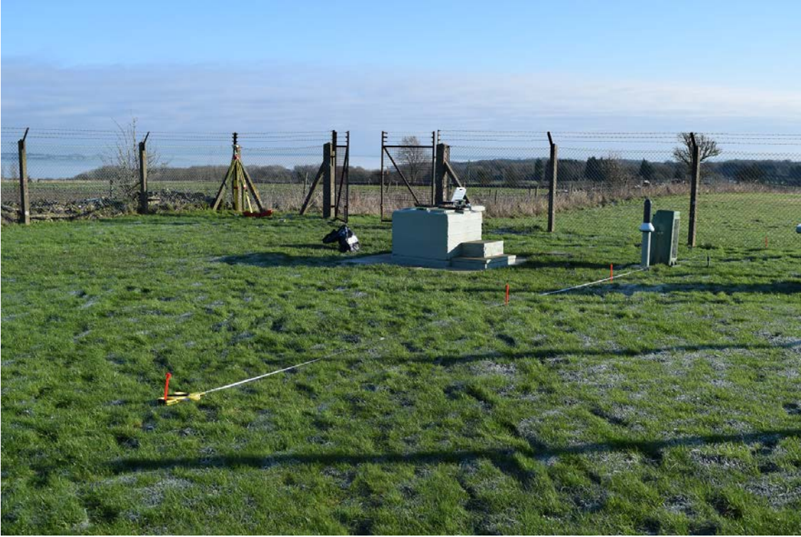
Figure A.4: Picture of the fenced off nuclear bunker site at Broadway tower. A line of gravity data was taken in a line parallel with the centre of the picture.
