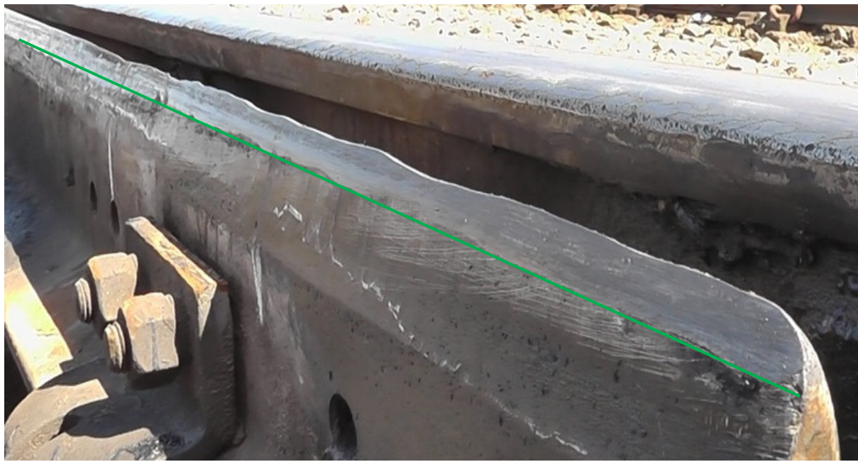
Figure 5-41 Example of damaged switch rail (photo 7)
