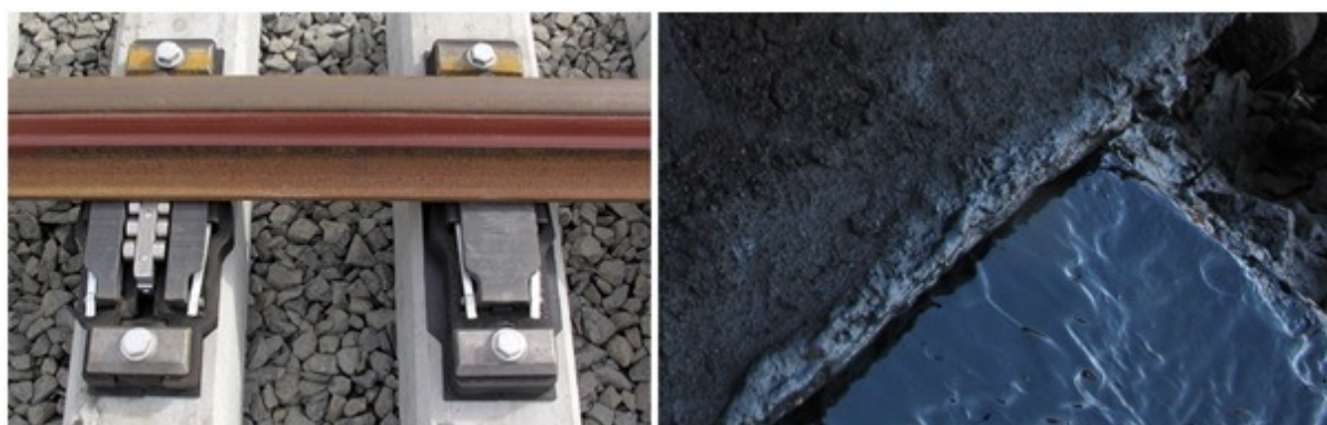
Figure 2-14 Voestalpine switch rollers (left); a heavy lubricated slidechair (right) left picture Courtesy and Copyright Voestalpine
