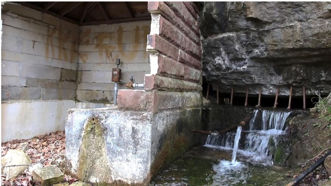
Figure 13: Graffiti in the pump house at Hammett Hill Spring, Warren County, KY
