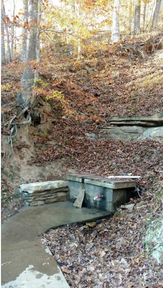
Figure 19: Briscoe Spring with bench and concrete pathway, built by Jeff Moser, Powell County, KY (photo provided by Jeff Moser)
