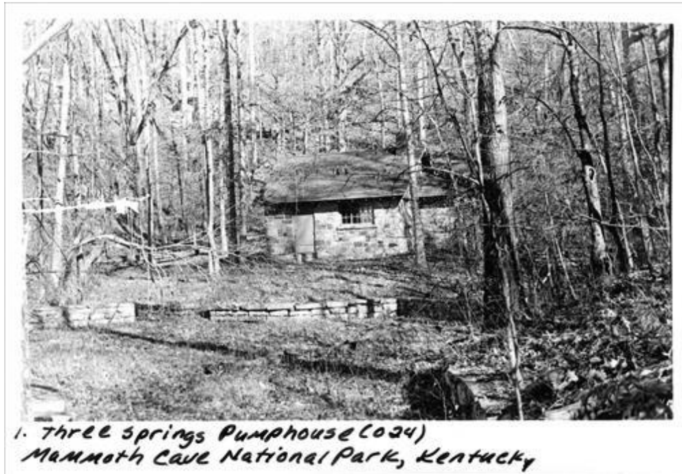
Figure 17: Three Springs Pumphouse, Mammoth Cave National Park, Mammoth Cave, KY (photo property of the National Park Service)
