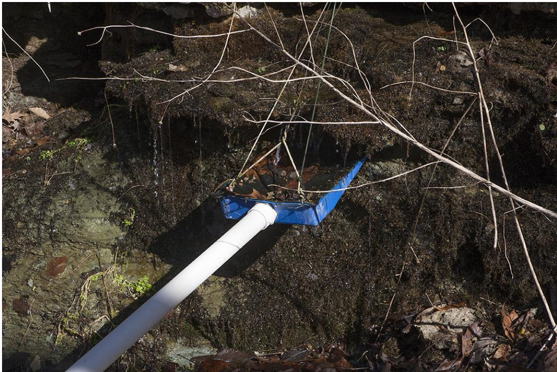
Figure 20: Spring filtering system, made with a paint tray and window screen, Cold Spring, Barren County, KY
