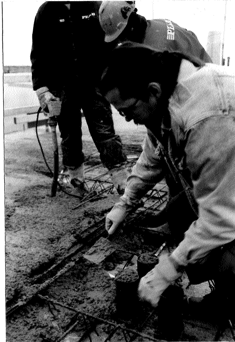
Fig. 4. Standard cylinders were fabricated on the building site [6].
