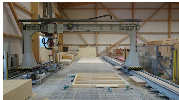
Figure 1 Woodworking gantry-robot cell at SMERobotics partner Mivelaz Techniques Bois SA, performing wall panel assembly for pre-fabrication houses and free-form milling.
