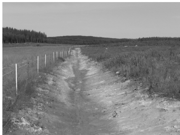
Figure 19. New Ditch on the Clearing, Farm CF 9
