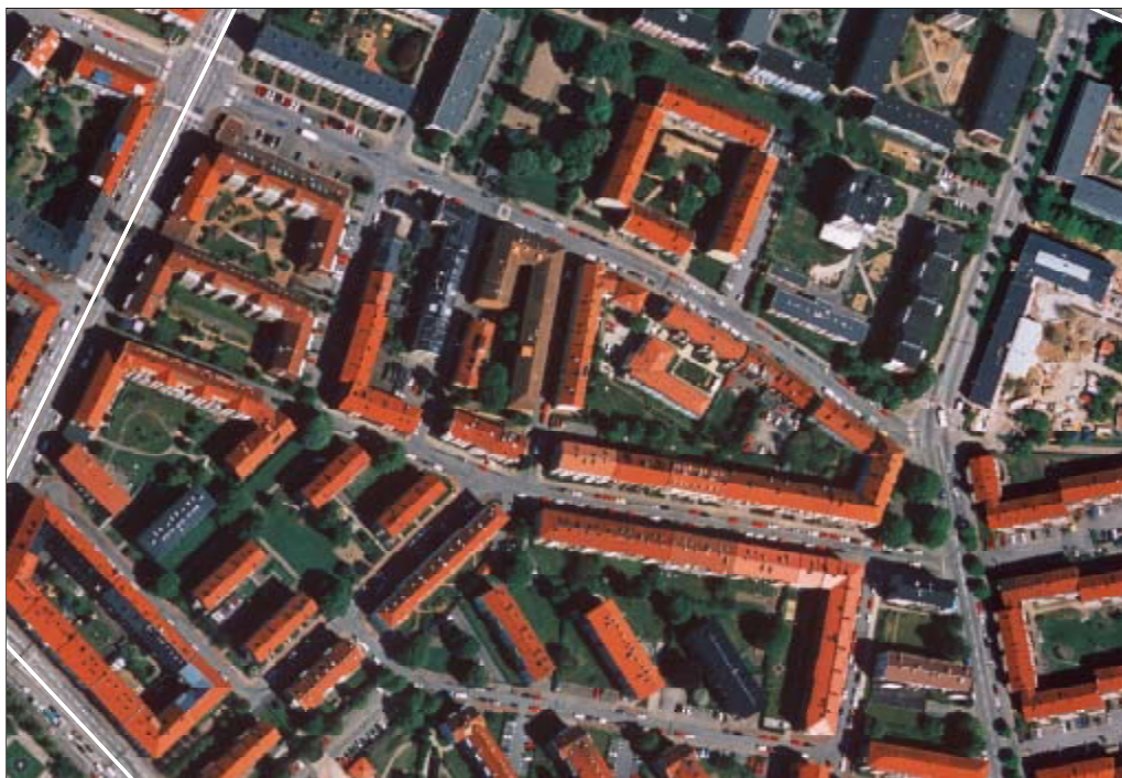
Figure i:20 The southern part of Östra Sorgenfri is dominated by the lamellar building in the grid, although several other super-morphs are present, such as the routescape and the closed grid block.
