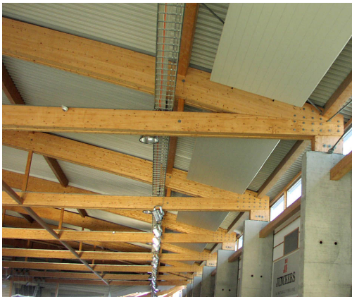
Roof before failure
