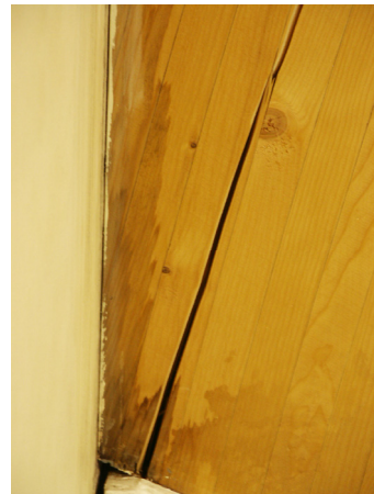
Figure 115-2. Crack at column fitting to the steel part.
