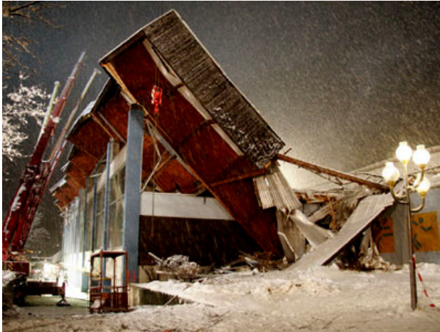
Fig. 1. Collapse of wooden roof for ice skating arena in Bad Reichenhall, Germany
