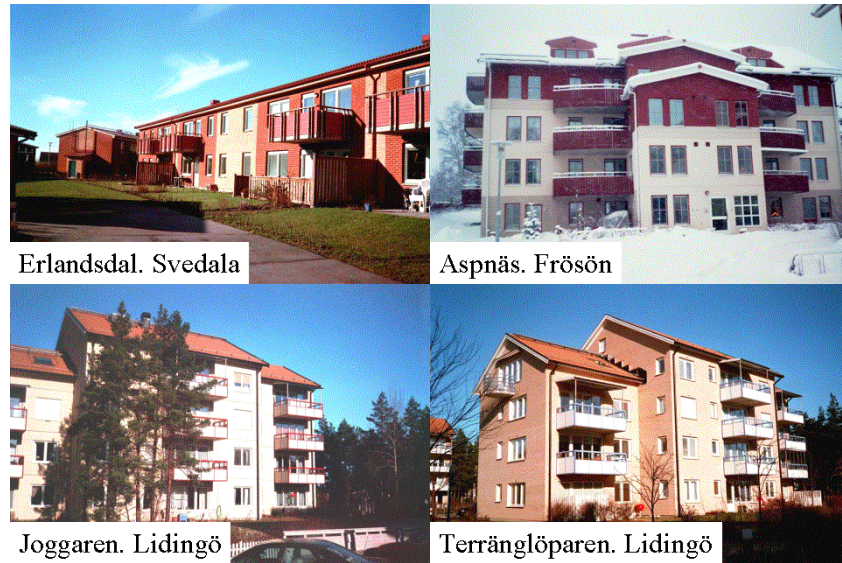
Figure 4.7 Buildings in case study on life cycle costs (Johansson and Öberg, 2001). Photos by the author.
