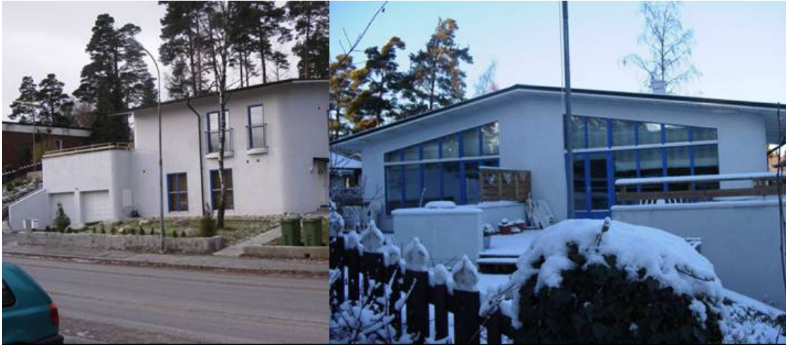
Figure 7.2 Example B. Façades towards the East and South. Photos with permission from the Maxit Group.
