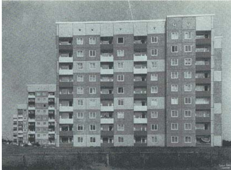
Figure 4.5 Early 1960s social mass-housing with prefabricated concrete elements.
