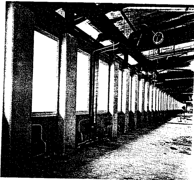
Fig. 11.1.8 a. Facade columns with fire insulation in the form of prefabricated gypsum plaster sections
