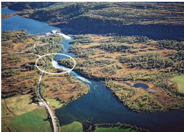
Fig. 1 Aerial photograph of the location of the embankment test facility in Røssåga river. In the upper left part is the Røssvatn reservoir impounded by the Røssvassdammen dam (from Høeg et al. 2004)
