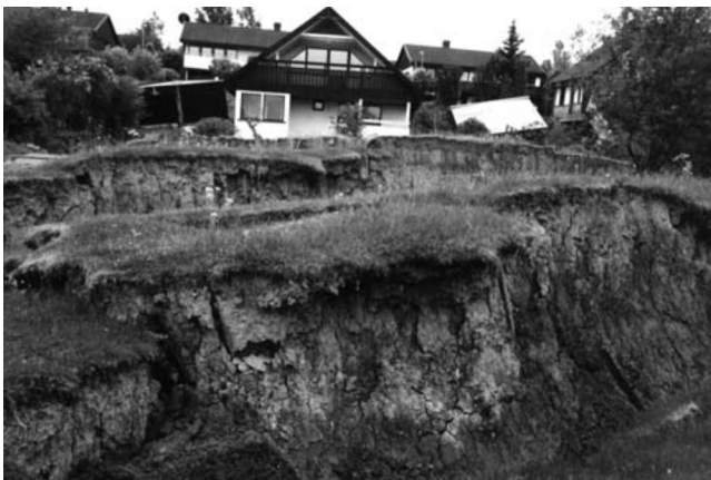
Fig. 7. Photograph of residential area in Vagnhäräd after slope failure within Trosa River Valley in 1997 (photographer: Jan Lindgren, Swedish Geotechnical Institute)
