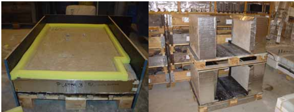
Figure 18. Left picture shows one floor construction in batch 1 prepared for screed application, one corner was spared for sample extraction. Right picture shows four floor constructions from batch 2 vertically tilted in climate conditioned room not yet covered with screed.
