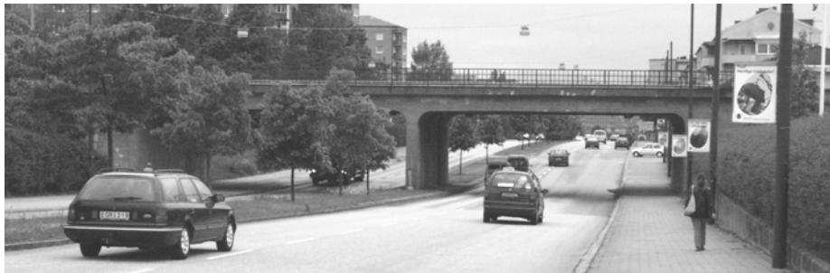
Figure 7.1 Photograph of the investigated bridge.
