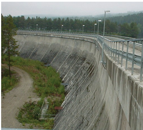
Figure 4-1 - Gravity dam at Stadsforsen.
