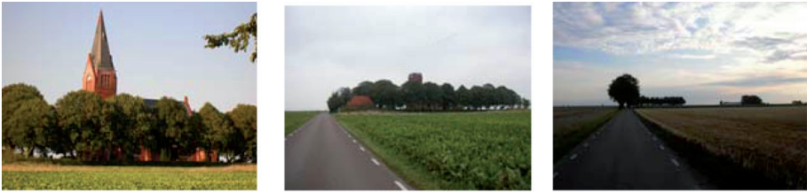
121.1 New Maglarp Church 2006 (left), during its demolition 2007 and the empty site in 2008 (right).
