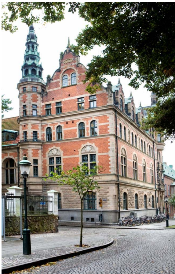
The IIIEE building in the centre of Lund
