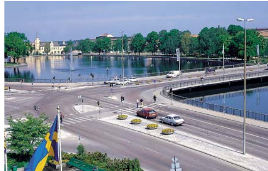
The major signalized intersection before the reconstruction.
