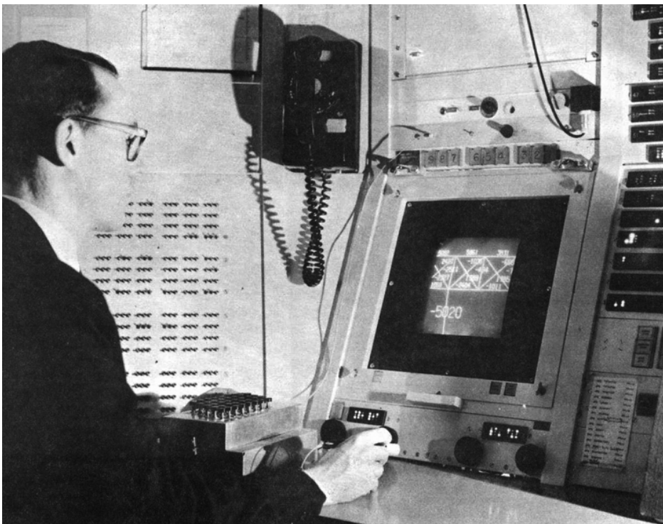
Figure 4.3: Sketchpad - the first CAD tool
