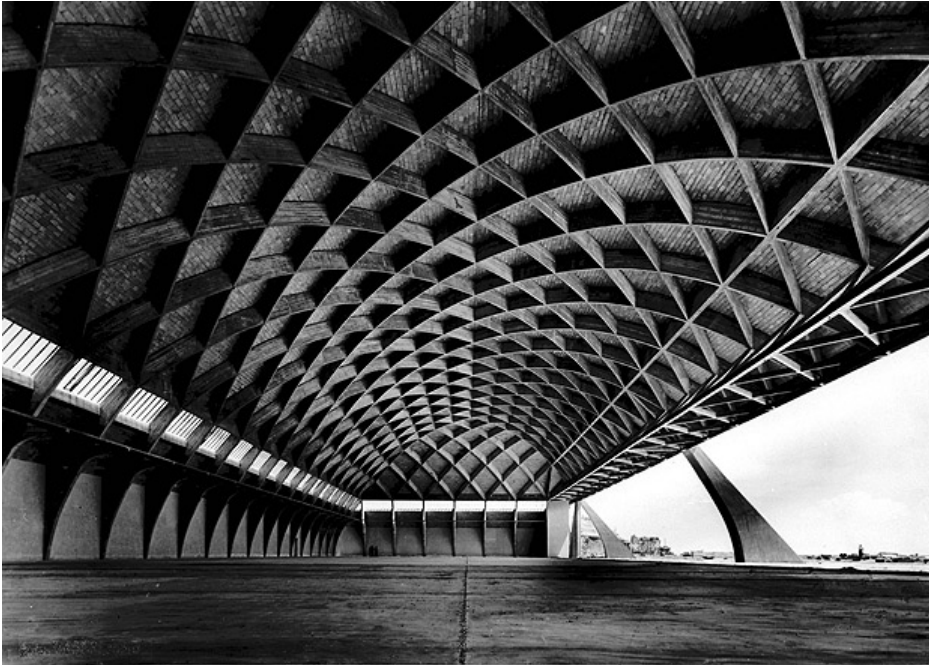
Figure 1.4: Pierre Luigi Nervi - Air hangar, built 1936
