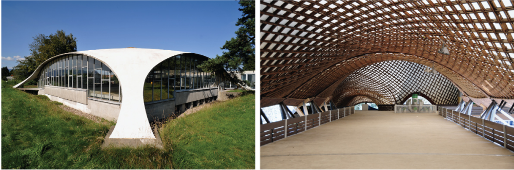
Figure 3.1: Example of form-found structures. Left: Concrete dome by Heinz Isler, © Chriusha, Wikimedia Commons; Right: Multihalle in Mannheim by Frei Otto © Hubert Berberich, Wikimedia Commons
