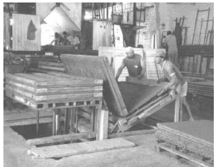
Fig. 18 Stripping 24 hour old slabs (Climatex, Brazil).
