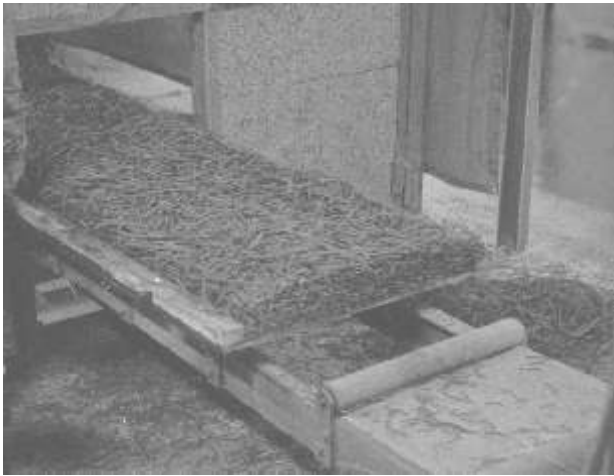
Fig. 2 Mould filled to overflowing with a mixture of wood-wool, cement and water before compressing (Tepro, Sweden).
