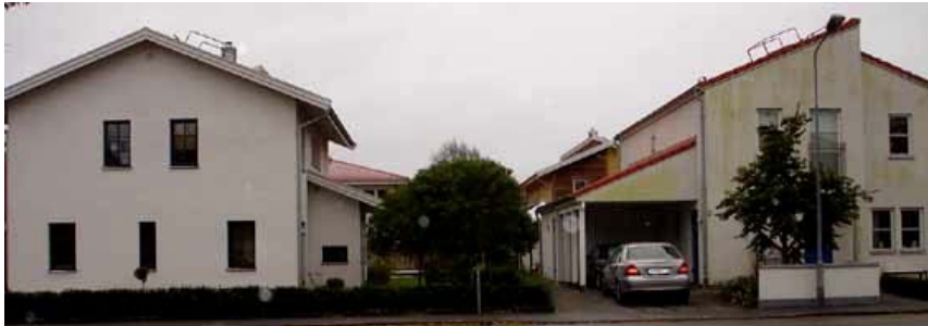
Figure 5.16 North-facing façades from two neighboring houses in Åkarp, built with same materials one month after each other in 2000. House 4 to the left, house 1 to the right
