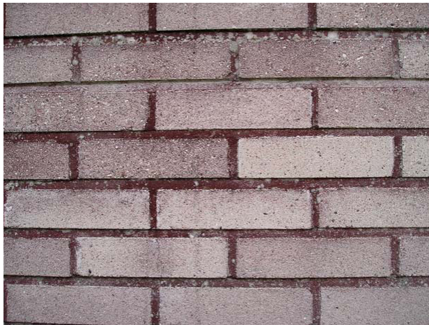
Figure 1 Coating of red green-algae on a masonry wall. Different lichen species can also be seen
