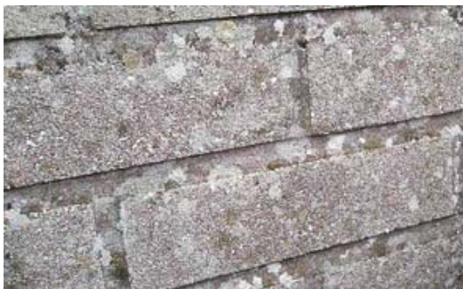
Figure 5.5 Calcium silicate brick wall with growth of several different organisms, mostly lichens
