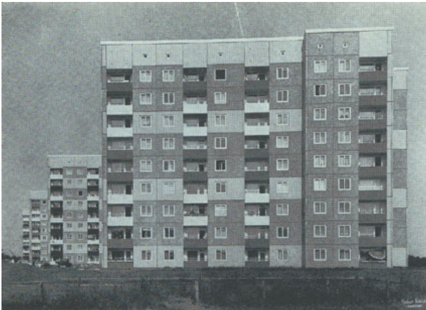
Figure 3.10 Early 1960s social housing with precast concrete
