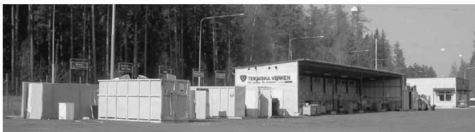
Fig. 2. Containers for bulky hazardous waste, cages for electric and electronic waste, and the area covered by a roof at Malmen Recycling Centre.
