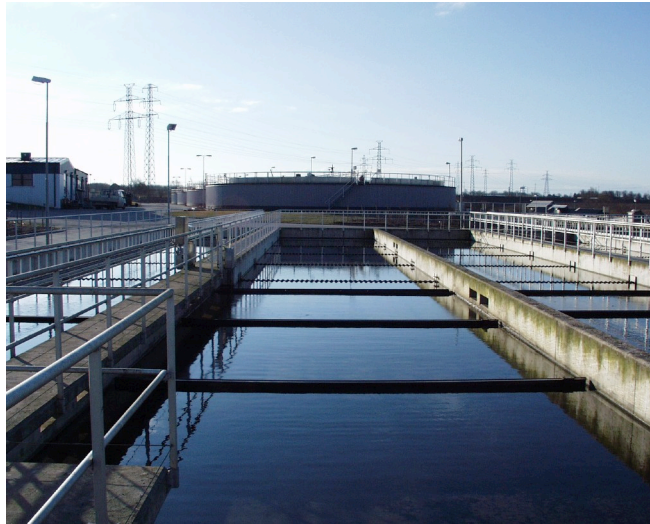
Figure 2.8 Settling basin at Källby treatment plant in Lund (Photo Michael Ljunggren).
