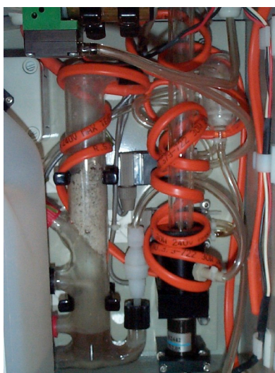
Figure 5.7 The glass reactor inside the on-line ammonia sensor from Awa Instrument, which is a part of the UV-pcx instrument.
