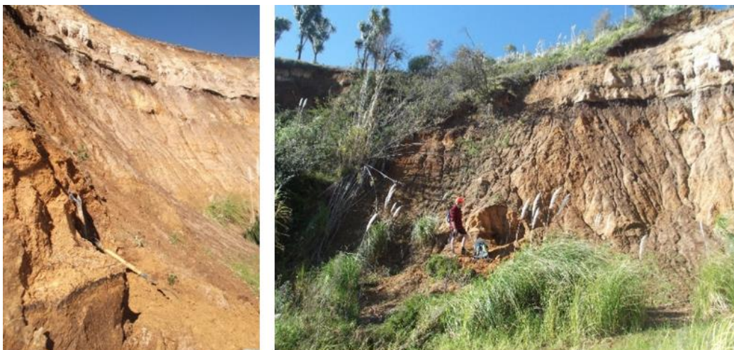
Figure 4.9. SS2 location on the failure scarp.
