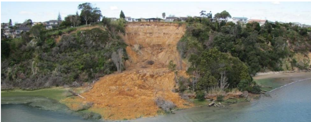
Figure 4.6. Bramley Drive failure viewed from the Harbour. Photo: Peter Clarke.
