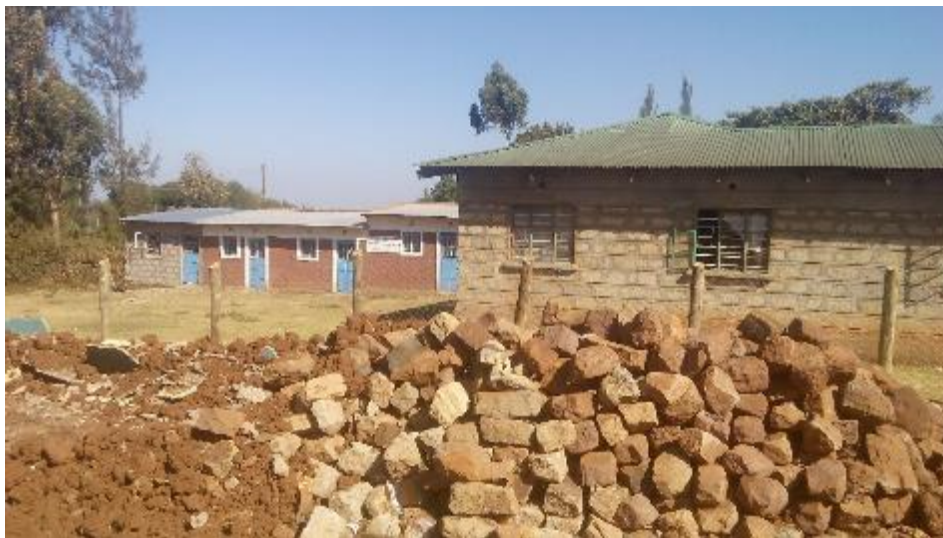
Plate II. Construction of Administration Police Lines in Uasin Gishu
