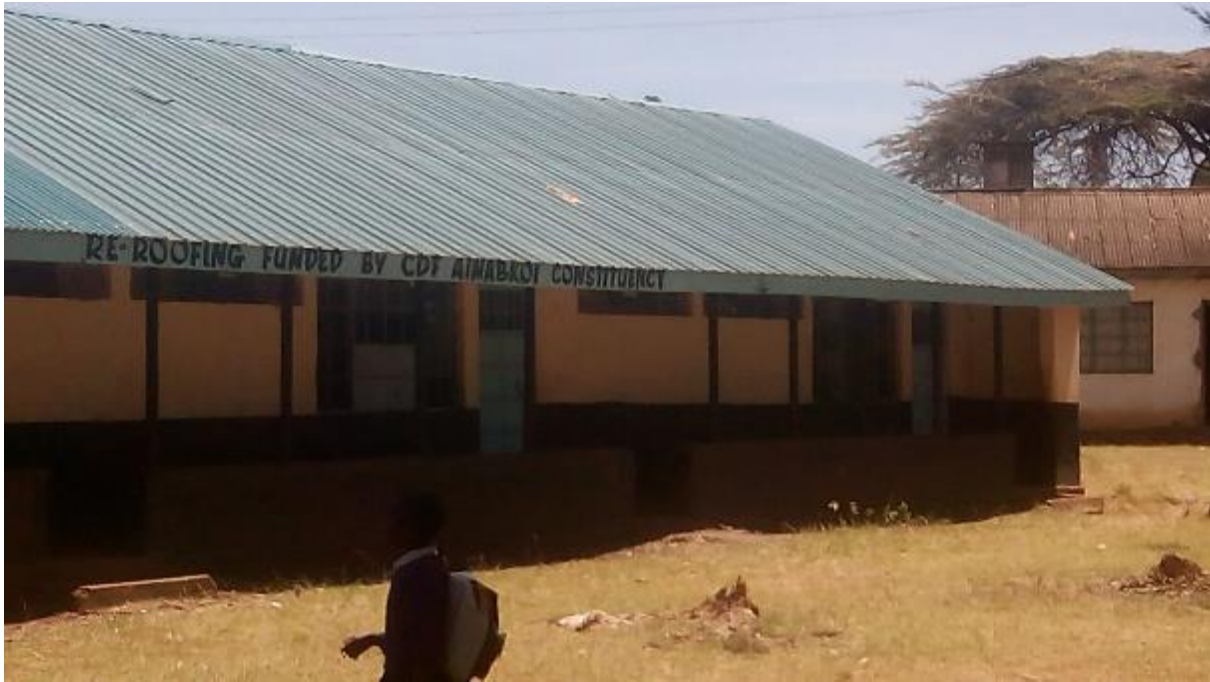
Plate III. School Construction in Uasin Gishu County
