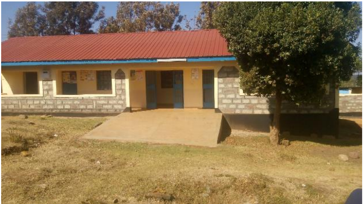
Plate IV. Construction of Shool Adminstration Block
