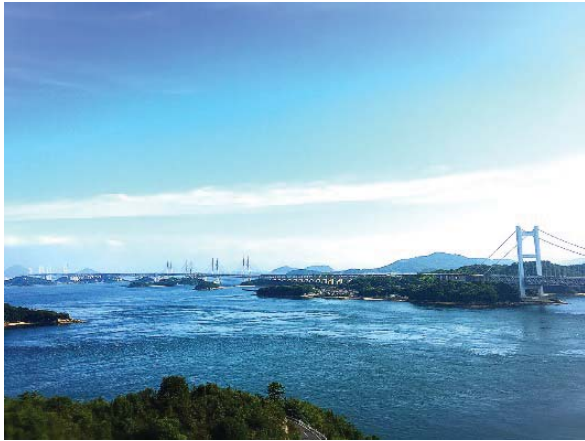
Fig. 15 The northern part of Bisan Seto Big Bridge (Seto-Ohashi) from Washuzan photographed by the author (July 17, 2016)
