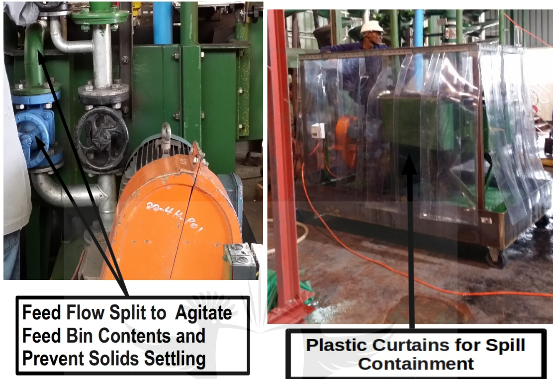
Figure 5.2: Agitation mechanism used to prevent solids settling in the feed bin
