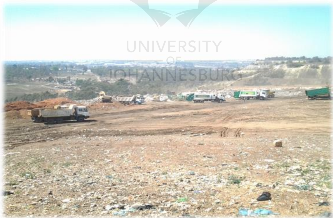
Figure 2: 5 : Landscape Overview of Marie Louise Landfill Site
