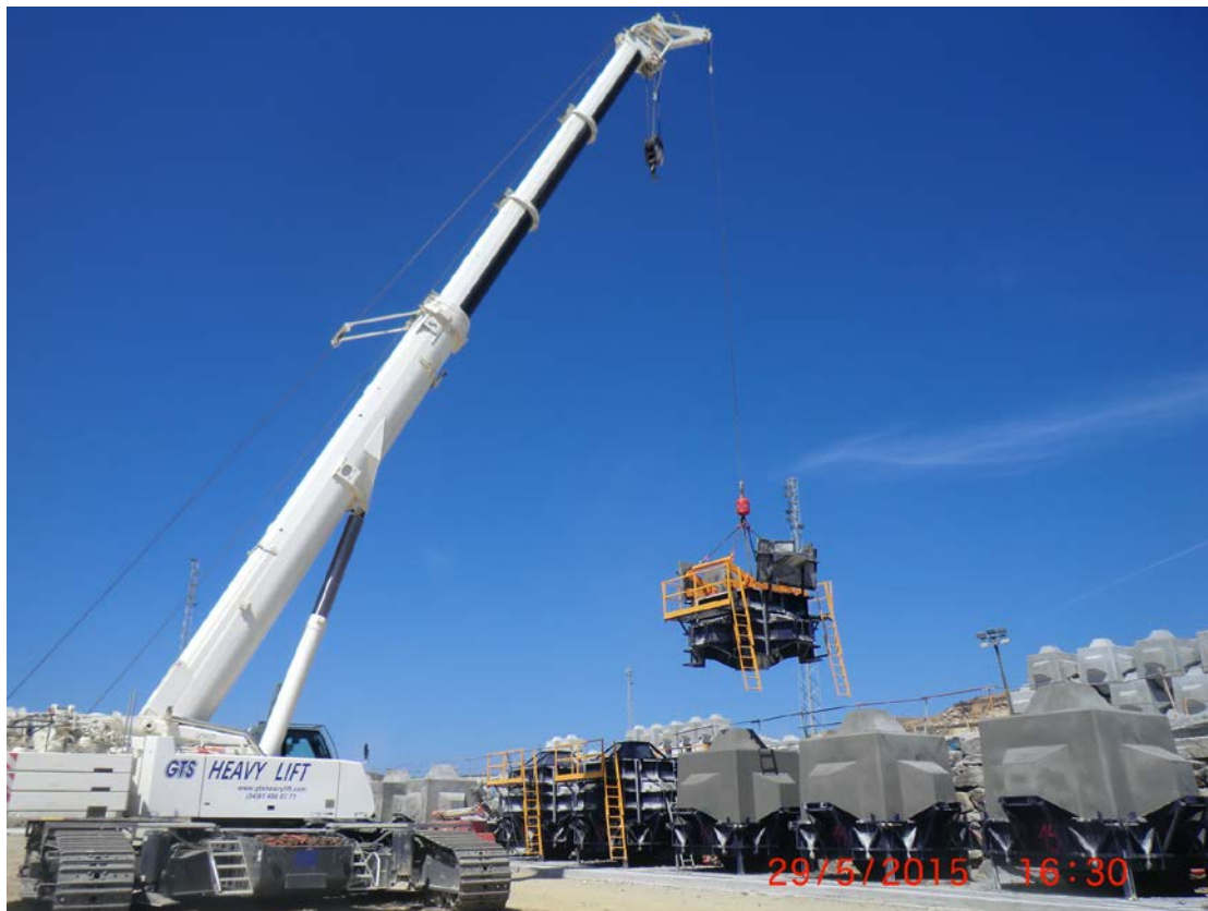
Figure 6. 45-tonne Cubipod ® formworks in the production line.
