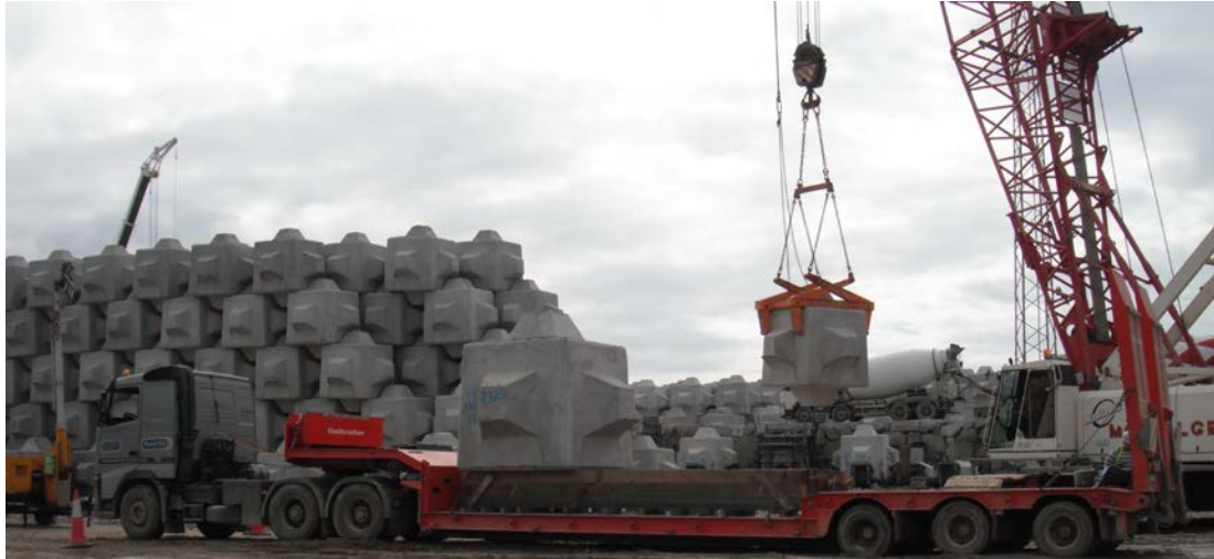
Figure 8. Loading Cubipods onto flat bed platform truck to be transported to the placement site.
