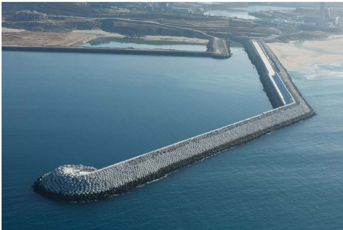
Figure 13. Western Breakwater (November 16 th , 2016).
