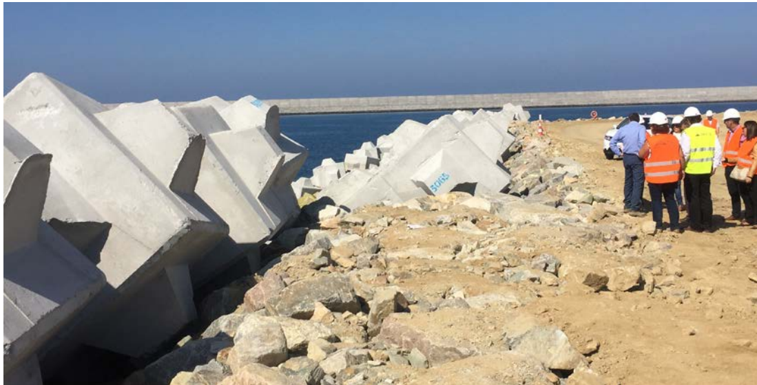
Figure 9. Transition from single-layer to double-layer 25-tonne Cubipod ® armor.
