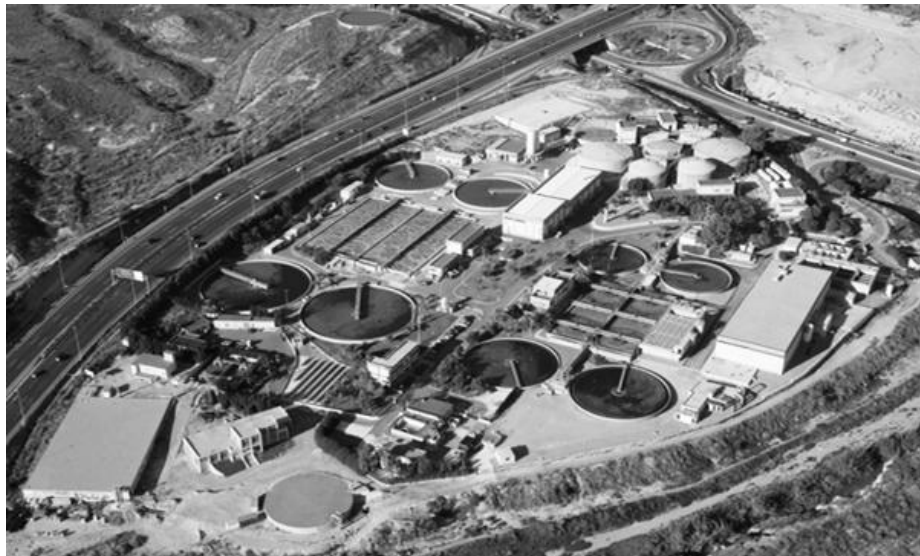
45 Figure 1. “Rincón de León” WWTP-WRP (EPSAR)
