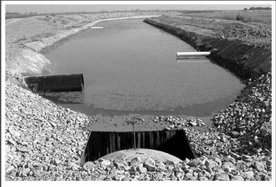
Figure 9. Grade-stabilization structure, water-control structure, and excavated storage reservoir.
