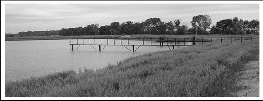
Figure 6. Irrigation storage reservoir.
