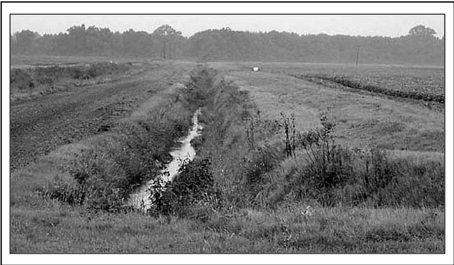
Figure 10. A surface drain.
