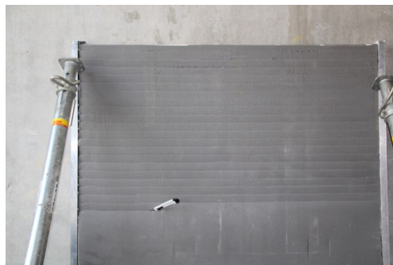
Figure 55 Application of the thermal insulation material at the window shutter
