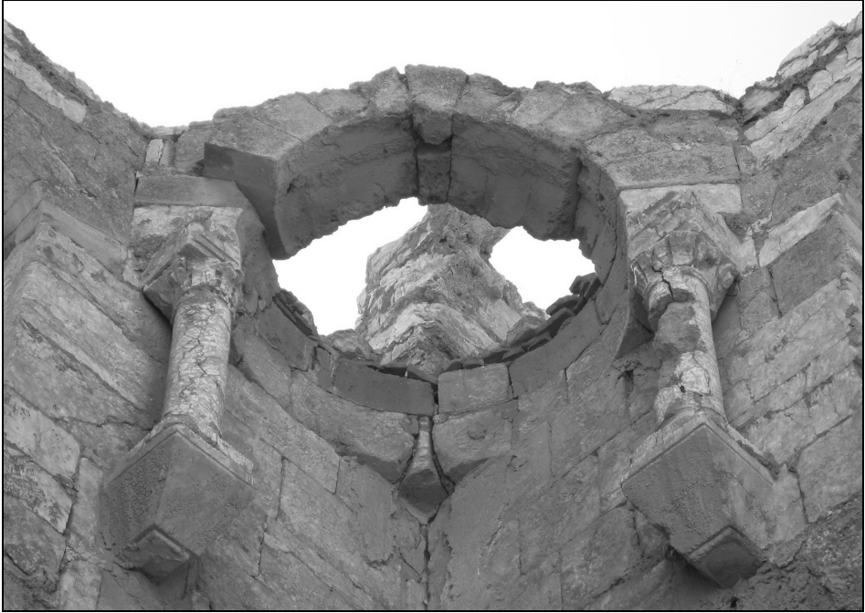
Fig. 8. Resafa, Church of the Holy Cross, "Eckbrücke" (photo: M. Bogisch).
