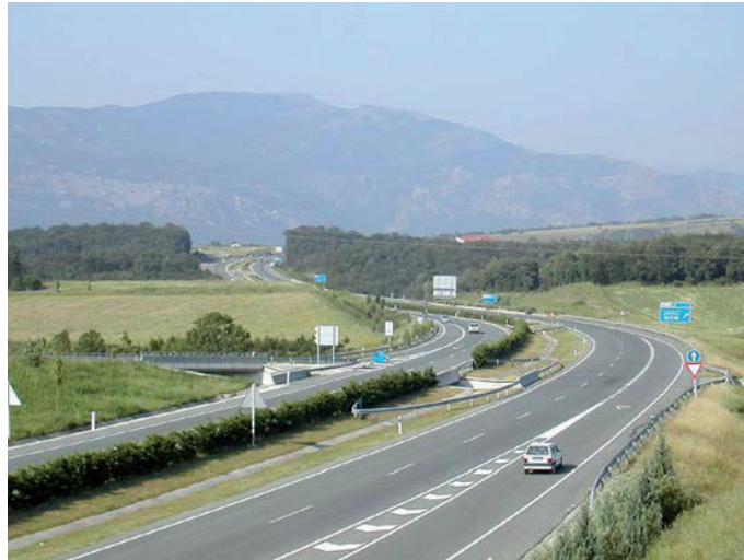
Figure 2. The photograph shows clearly how the A-10 motorway crosses one of the remaining forested patches, stretching across the gap between the Aralar and Urbasa-Andia mountain sides. Photographer: Luis Sanz Azcarate.
