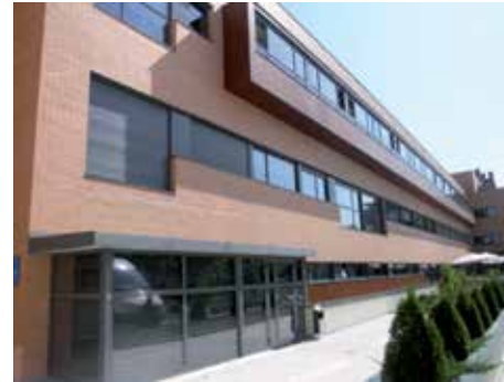
At the Laguna Care Center, Madrid (Spain), there are two PCUs and several other services such as a daycare centre, a nursing unit, a respite unit, rooms for the home care team and an education centre for healthcare professionals, relatives of patients and volunteers.
