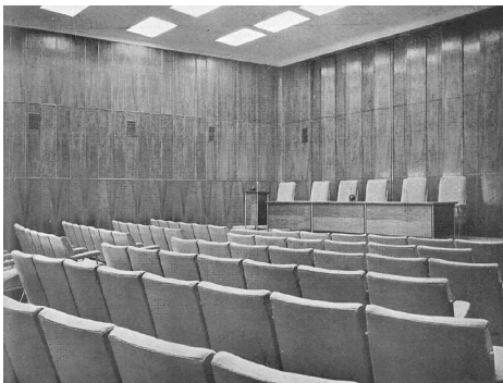
Figure 9. Impulsion and return vents in the conference hall. Image from 'Informes de la Construcción'
