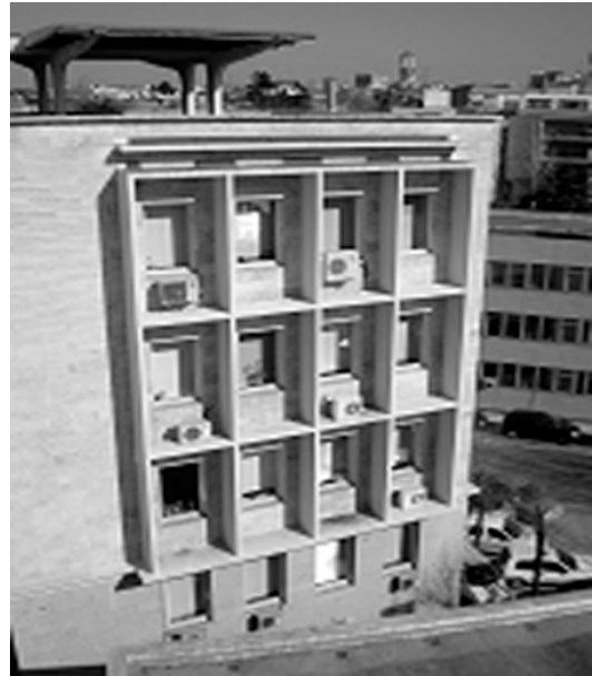
Figure 4. The photograph shows how the brissoleils barely shade the windows, although we must take into account the fact that the photo was taken at midday in February when, thermally, the sun should shine into the building
