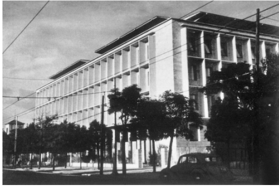
Figure 1. Exterior view of the Juan de la Cierva Trust Building
