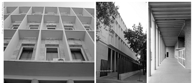
Figure 2. Images of the exterior and the entrance portico
