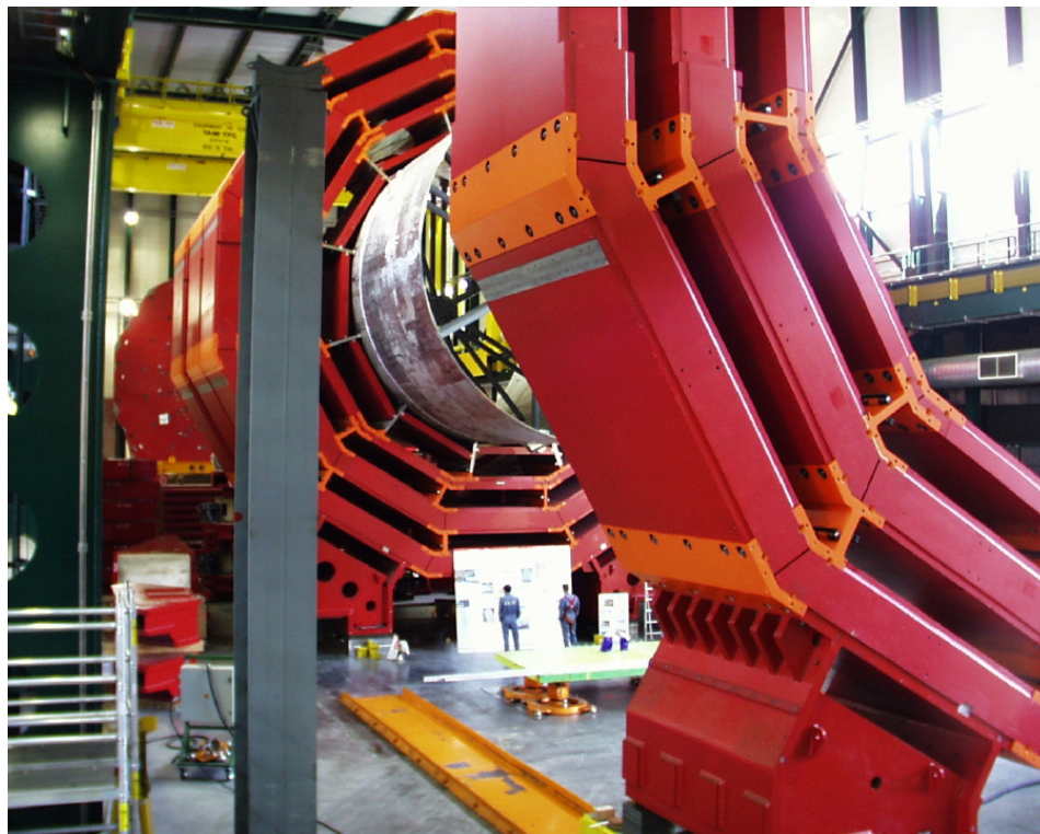
Figure 5.4: A photograph of the steel-yoke in the early stages of assembly. The centermost wheel in the barrel support the superconducting coil. One of the endcaps yoke can be seen at the back.
