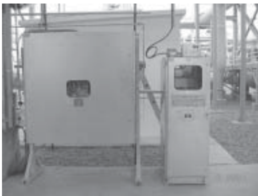
Figure 4. Photograph of online system for Hg in natural gas
