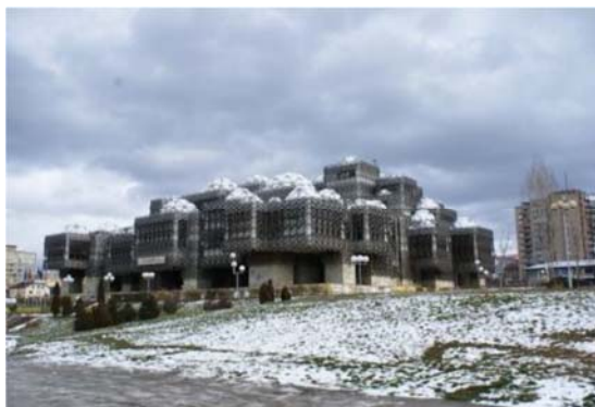
Fig. 2. View from the surroundings showing cubical volumes and domes, (photo: Eris Kajtazi)
