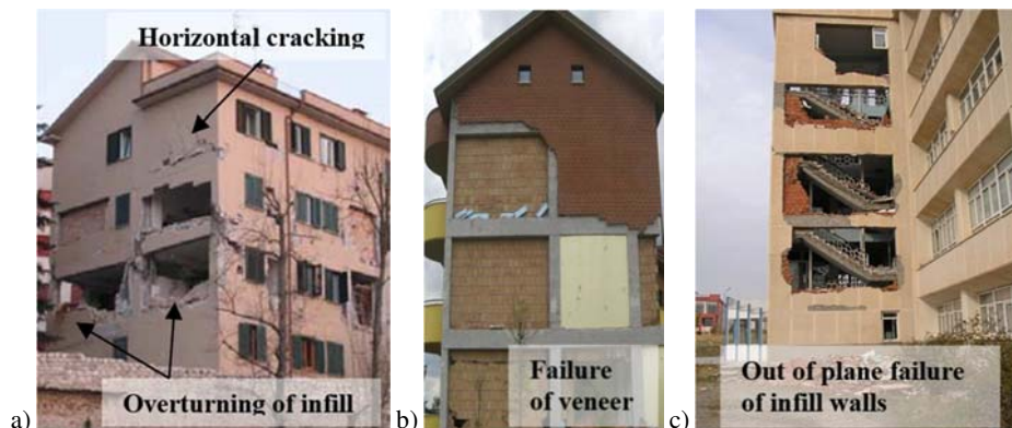
Fig. 3. Out of plane overturning of masonry infill, a) Abruzzo earthquake (after Morandi et al. 2013); b) Failure of veneer, Abruzzo (after Vicente et al. 2010); c) Van earthquake [10]
