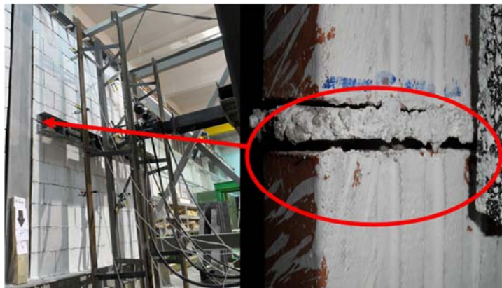
Fig. 8. Opening of horizontal crack in MW1
