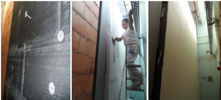
Fig. 10. Construction process of infill specimen MW2
