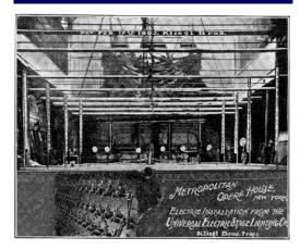
Metropolitan Opera's (1903) new electrical system from the 1913 Kliegl Brothers catalogue. There are eight sets of border lights above, four sets of wing lights, seven bunch lights upstage, and the switch board is located in the basement. X The image part with relationship ID rld3 was not found in the file.
