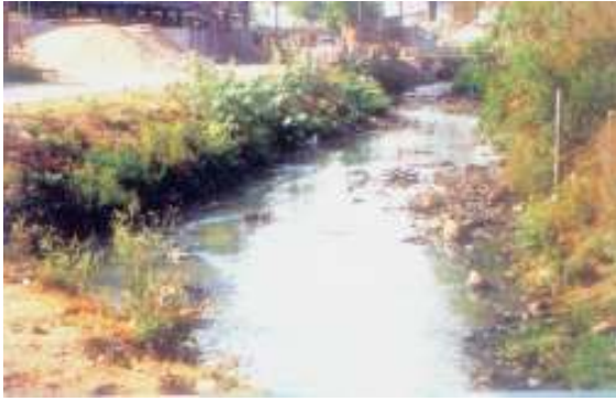
Fig 5. Disposal of untreated domestic sewage
