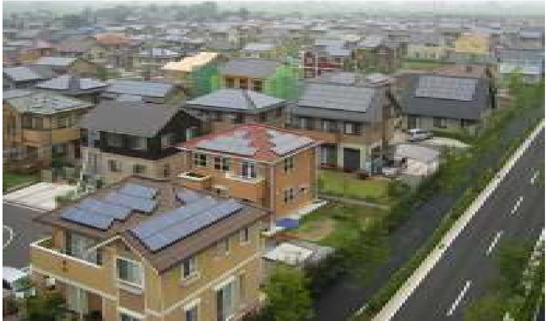
Figure 7. Japanese homes with PV arrays facing east, south and west in Ota City (Source : NEDO Official Homepage at www.nedo.go.jp )
