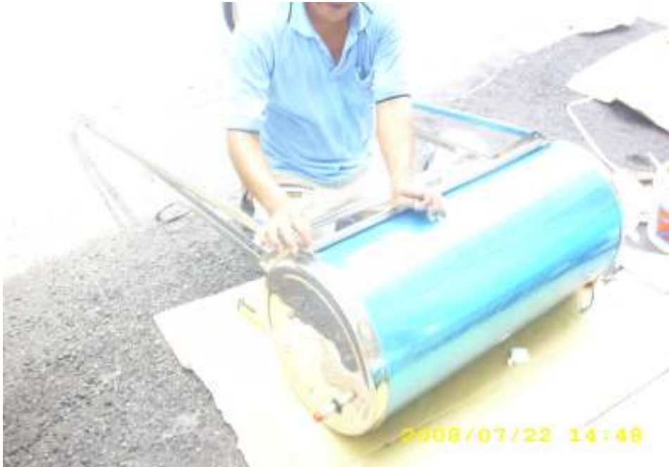
Figure 2.0 : Installation of the solar heater system parts in progress
