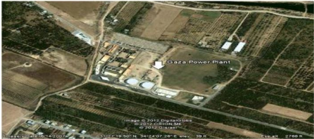
Fig. (1) Gaza power plant location from Google Earth.
